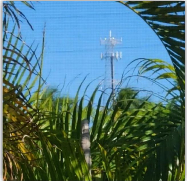
Cell Tower From Screened Deck (Zoomed)
